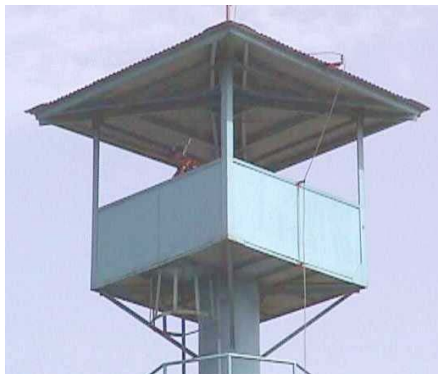
Photo 15.3. – Perimeter Security Tower
