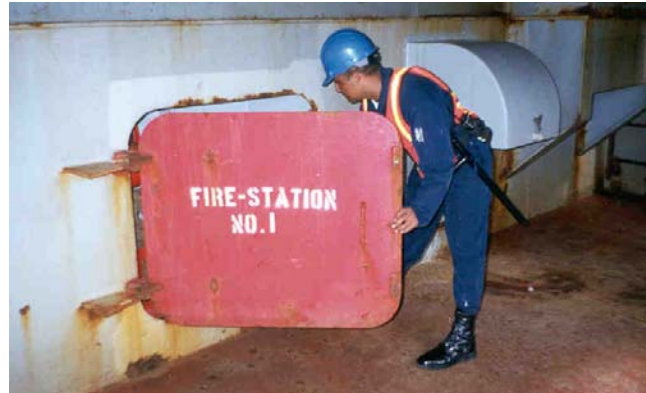
Photo 15.14. – Inspect the interior of fire hose boxes, storage areas, and cranes
